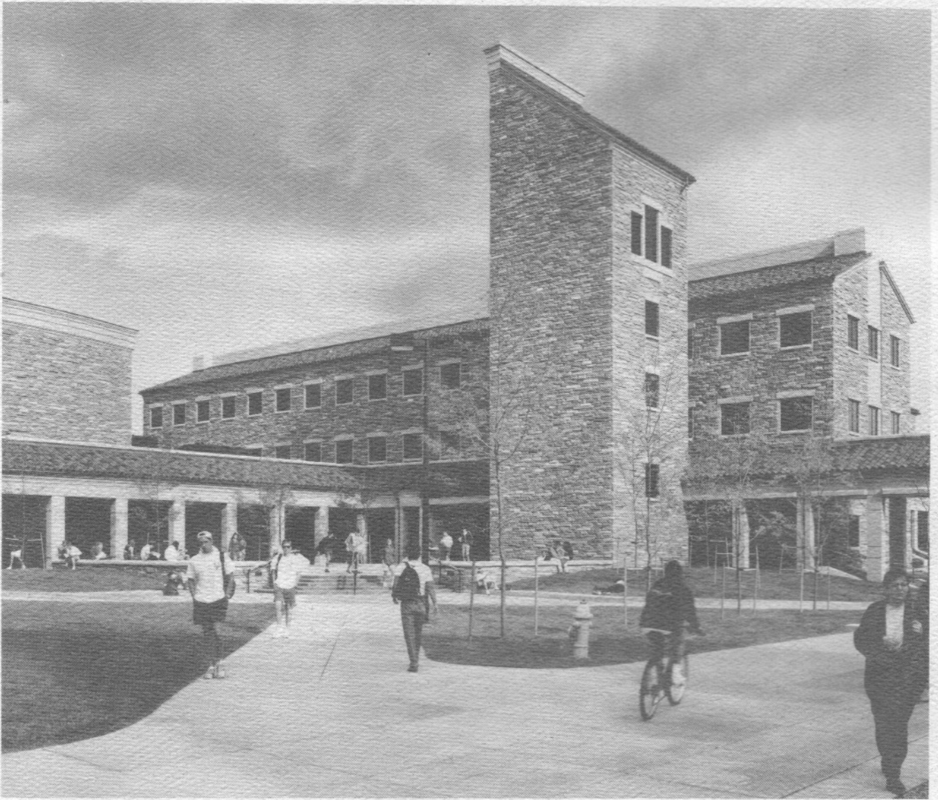
The Mathematics Building is located on Colorado Avenue, at the southern end of Folsom Street and adjacent to the Engineering Center on the west. The above photo faces a northwest direction. The lecture hall (MATH 100) is at the far left; the Gemmill Engineering Library is on ground and sub-ground levels in center; the Math Module Facilities containing a self-paced learning lab are ground level right; Mathematics Department offices are on levels 2 and 3, center and right.
